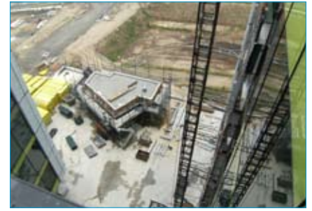
Café construction viewed from rooftop
