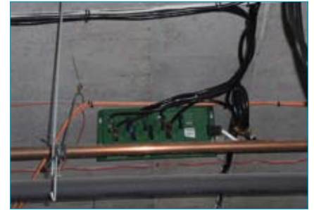
Data, lights and install of programmable lighting controllers in progress
