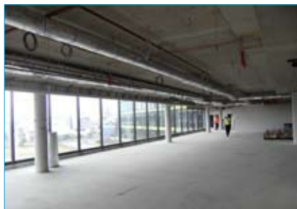
Areas ready for office fit out
