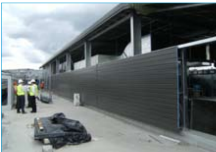
Rooftop plant under construction
