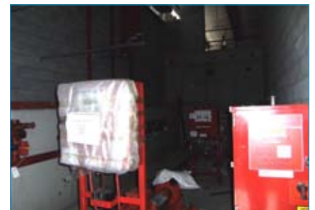
Fire system pumps and controls installation in progress
