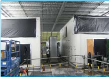
Air conditioning plant positioned and ductwork connection in progress
